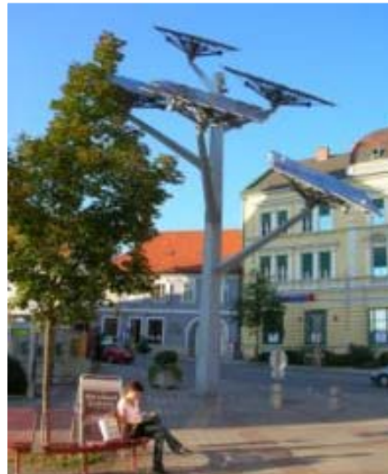
Figure 2. Solar "tree" placed out in the open where sunshine is abundant, Styria, Austria.
